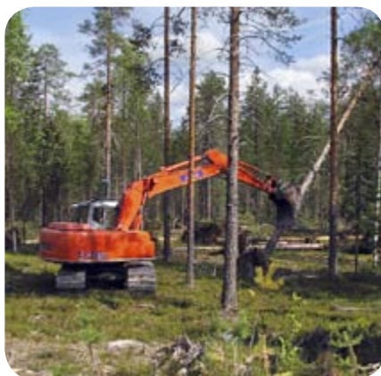
Figure 15. Dead trees felled with excavators resemble windthrown trees. PHOTO: JUHA SIEKKINEN.
