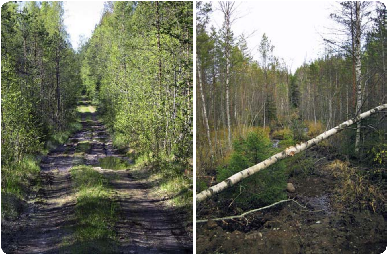
Figure 23. A forest road before and after measures taken to remove its traces from the forest landscape. The line of the road has been landscaped by shifting spruce and alder seedlings onto the road bed using an excavator. Trees moved in this way often successfully take root. PHOTOS: HELENA LUNDÉN.
