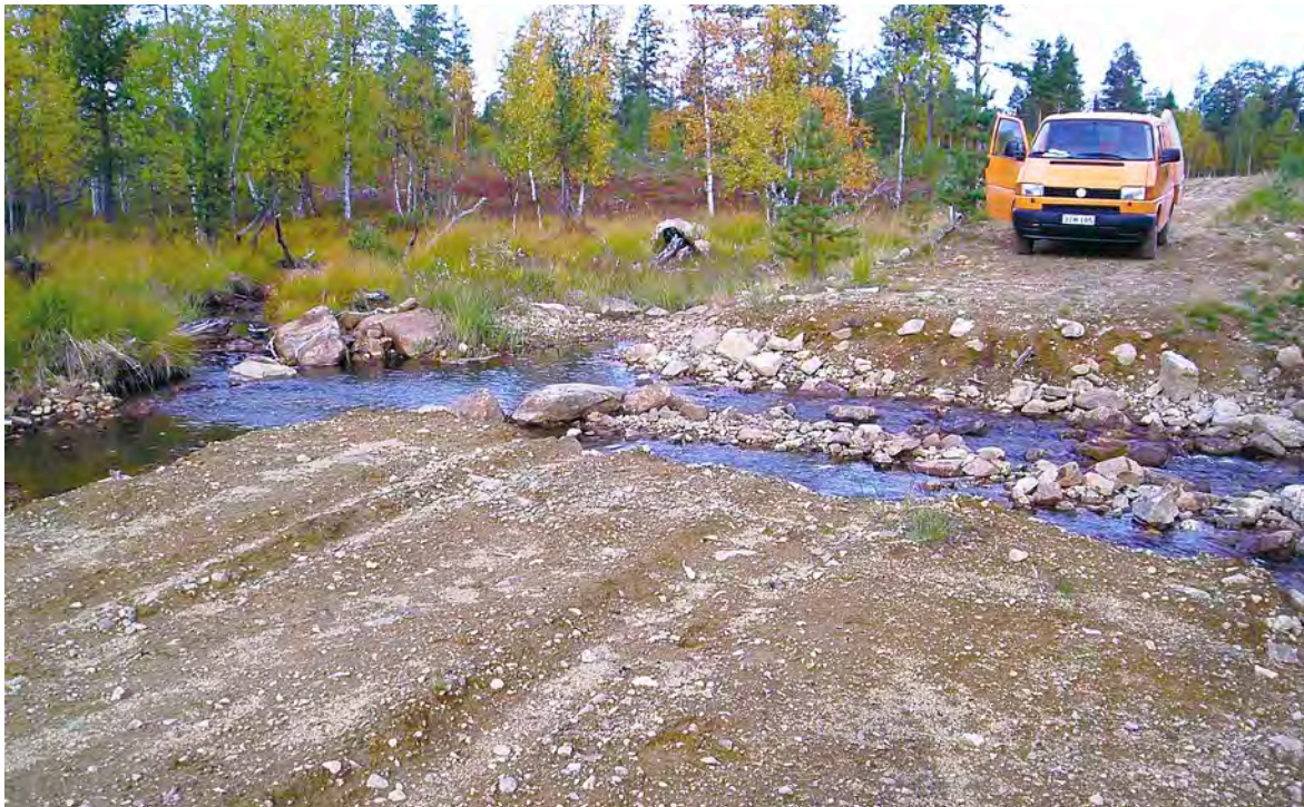
Figure 47. Forest road has collapsed into the river at River Hanhioja. Juvenile mussels were not detected below this site although they were abundant just above. Photo Panu Oulasvirta, Metsähallitus.
