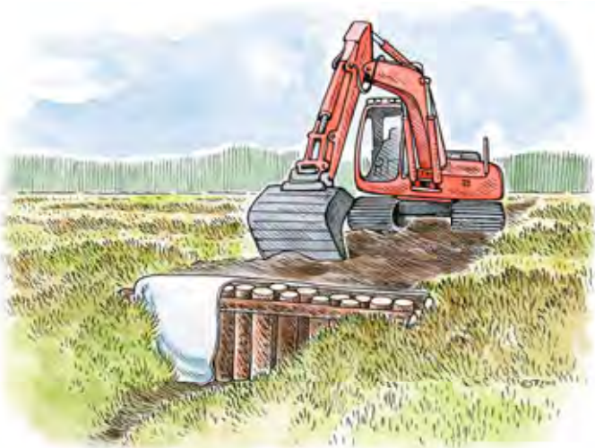
Figure 36. Log dams may be constructed where suitable logs can be cut from trees felled on the site. The top ends of the logs should stand out clearly above the level of the ditch banks. If the peat is deep, the logs can be sunk vertically into the peat, but where peat deposits are only shallow the logs can be put in place horizontally. The dam should then be covered with geotextile and peat. Log dams can be further stabilised with the help of supporting logs aligned at right angles to the other logs. ILLUSTRATIONS: TUPU VUORINEN.
