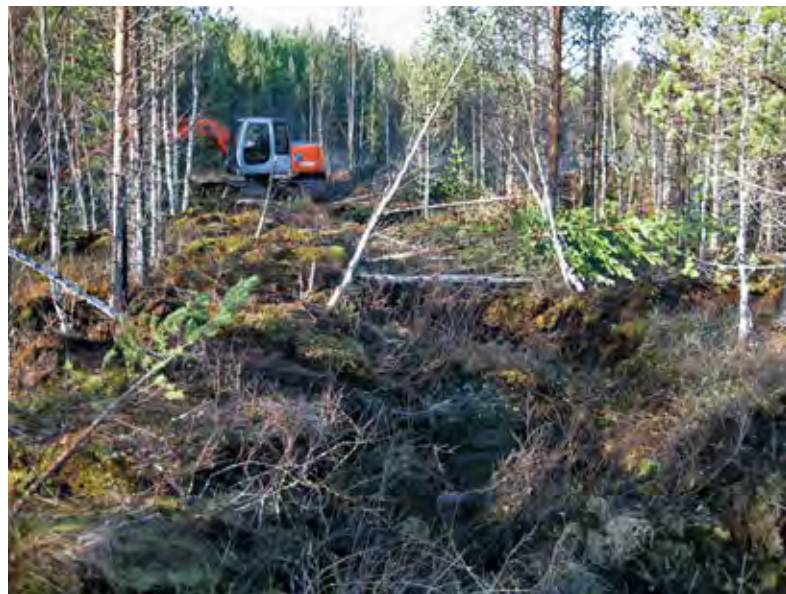
Figure 76. An excavator building a long dam in the main ditch in the drained area north of Vuosiaissalo, October 2009. By the excavator the ditch is near the boundary of an adjoining area with mineral soil. The forest behind the excavator is part of Vuosiaissalo. The water flows from right to left. PHOTO: REIJO HOKKANEN.
