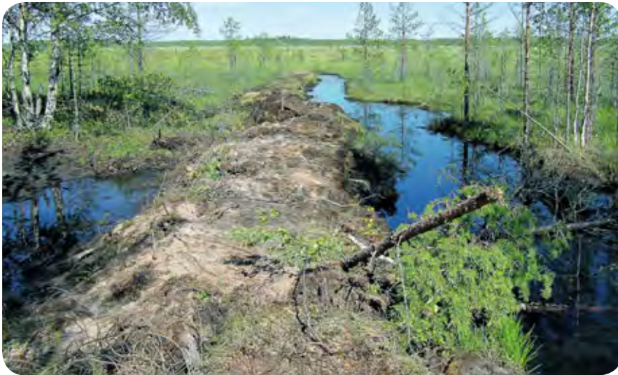
Figure 33. It may be worth making very long peat embankments in key locations with regard to water flows. In this site embankments were about 60 metres long. The dimensions of the embankments were clearly marked in the field with ribbons to ensure that the excavator driver made them long enough. This photograph was taken from the site of the infilled ditch, where water earlier flowed from right to left. The embankment was made perpendicular to the ditch line. A channel formed where peat was dug up to make the embankment, and water now flows along this channel to feed areas of flark fen which had not been drained but had nevertheless dried out. PHOTO: REIJO HOKKANEN.
