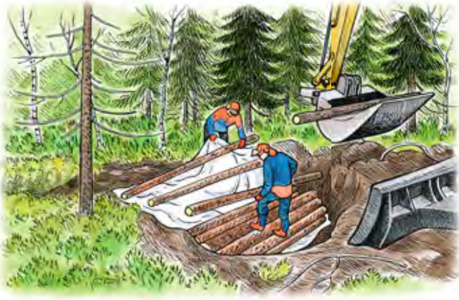
Figure 37. Obliquely aligned log dams can be made by combining manual and mechanical work, though an excavator driver can often make a dam alone if suitable logs are available. The site for the dam is first excavated. It should be wider and deeper than the ditch for improved stability. Excavated peat and ditch spoil is then used to construct a diagonally profiled banked dam that rises above the level of the surrounding peatland. Log supports are then laid horizontally over the entire height of the banked dam. Geotextile can be laid down on top of or beneath the logs. In the illustrated example the direction of water flow is right to left. This kind of dam is suitable for almost all restoration sites in wooded peatlands. ILLUSTRATION: TUPU VUORINEN.
