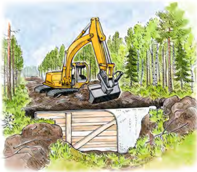
Figure 35. Tongue-and-groove boards can be used to help make dams in large or badly eroded ditches. The geotextile used to cover the boards is only partly shown in these illustrations to enable their underlying structures to be seen. Illustrations: Tupu Vuorinen.
