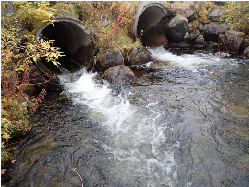
Figure 194. Culvert pipes under a private road in Vuohččojohka may prevent salmon parr ascending into the river. Photo: Aune Veersalu.
