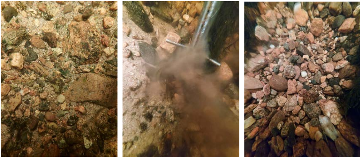
Figures 20. Restoration with Hartijoki method, same place before and after the treatment. Photos: Pirkko-Liisa Luhta.
