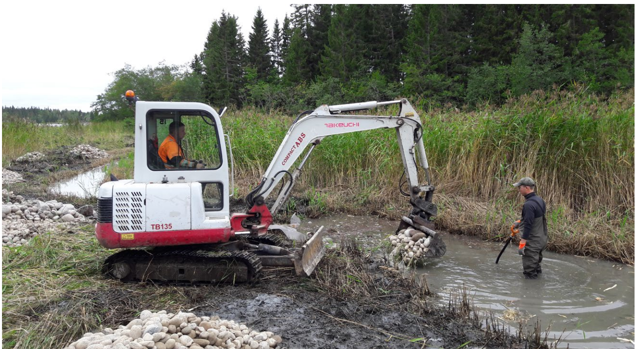
Figure 38. Stones are laid on the bottom of the channel to prevent rapid recolonisation by reeds. Photo: Sanna Kuningas/Natural Resources Institute Finland.
