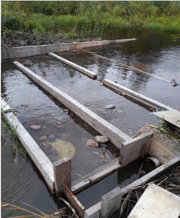
Figure 36. A fishway leading to a gloe lake helps fish migrate to their spawning grounds in the spring. Photo: Sanna Kuningas/Natural Resources Institute Finland.
