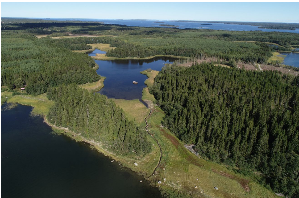
Figure 41. Backfladan and its restored channel after clearing of reeds. Photo: Lari Veneranta/Natural Resources Institute Finland.
