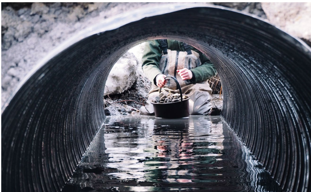
Figure 19. The culvert was installed deeper into the ground and filled with gravel and stones to create a channel extension that was as natural as possible. Photo of Verkvikfladan: Maija Haukkala/Metsähallitus 2019.
