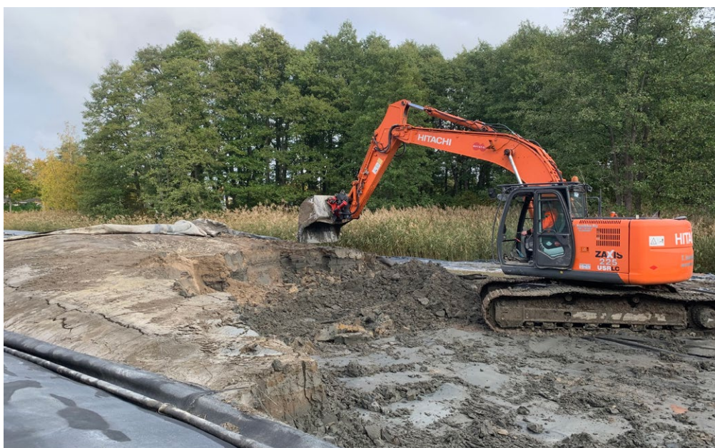
Figure 12. Dredged spoil that has solidified within a geotube. Depending on its properties, the spoil can be used in landscaping and for other similar purposes. Photo: Harri Huuho/MeriHamina Association.
